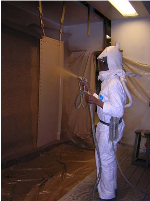
Performance Urethane Exterior Topcoat Application
